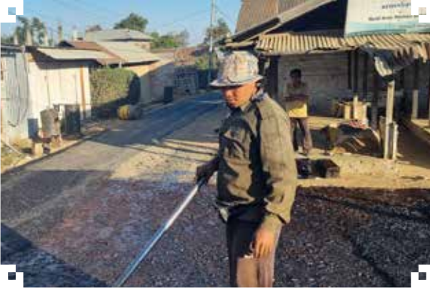
Blacktopping of Bishnupur Ward No 7 road. Enhancing connectivity
