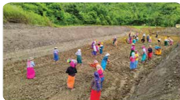
Construction of Public Pond at Kangyambem Lokchao maning leikai ward no.6 (2022-23)
