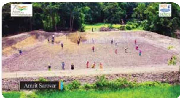
Construction of public pond at Chandrakhong Awang Leikai, Ward No. 9 (2022-23)
